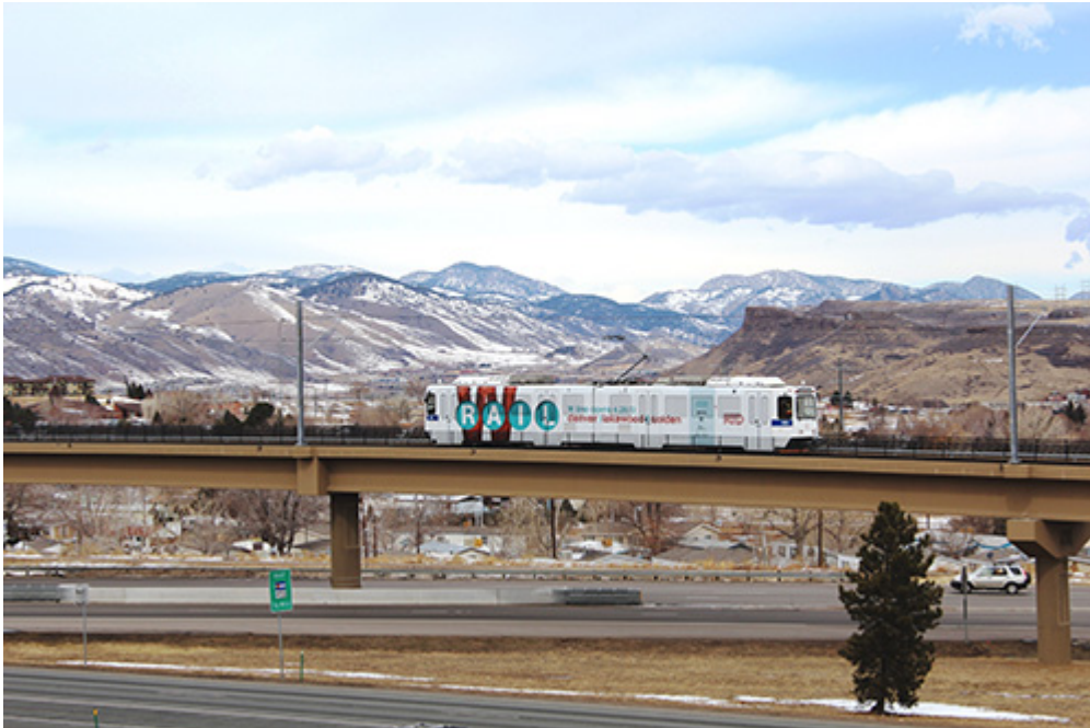
W Line Trains undergoing testing on the westbound approach to Jefferson County Government Center
